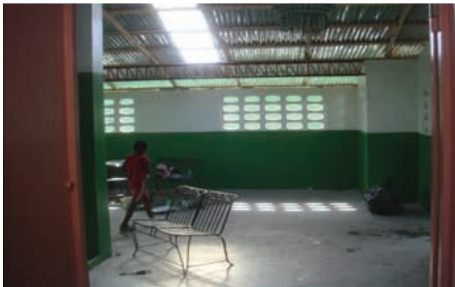
Part of the new roof with skylights that was put on in July by the work team
